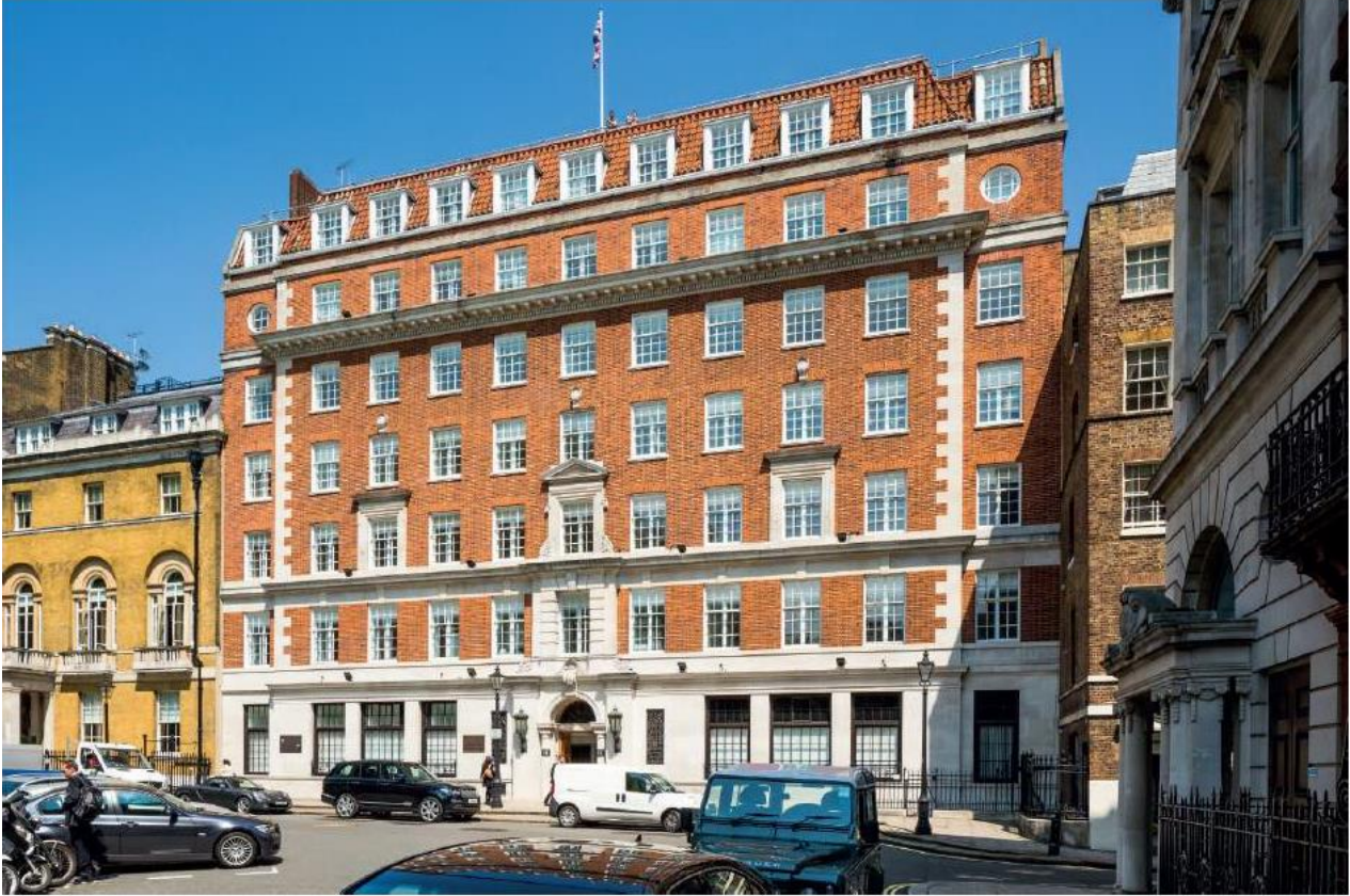
Existing elevation on to St James's Square
