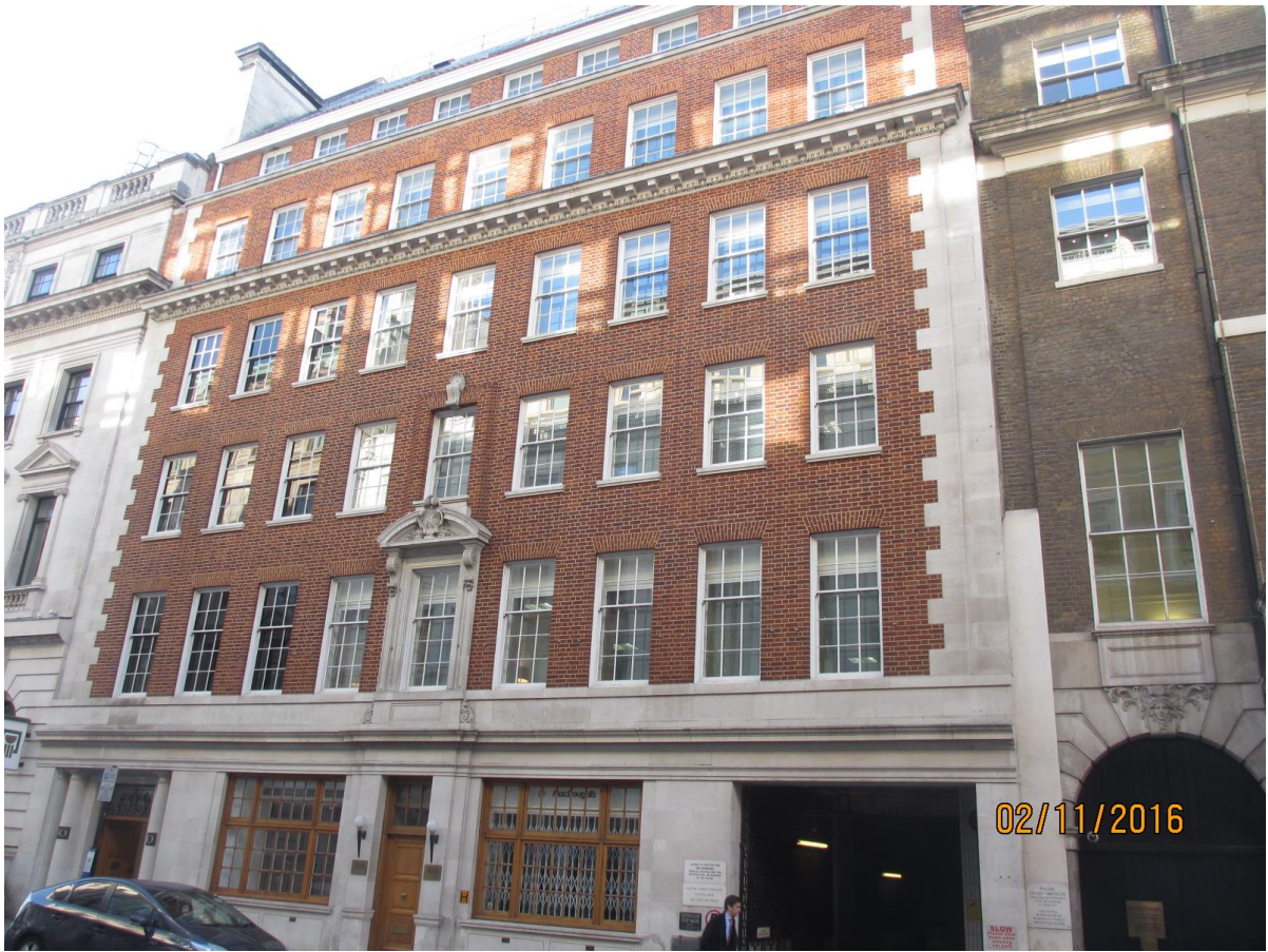
Norfolk House – elevation onto Charles II Street
